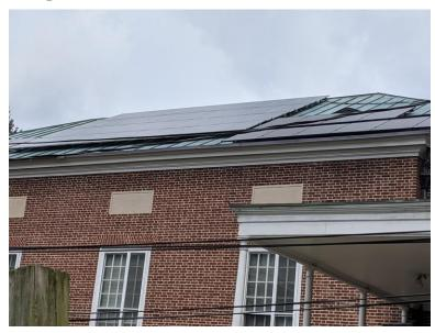
The Meetinghouse now has 52 solar panels, half installed in 2010 and the other half this summer of 2020. The new panels more than double the array's potential for producing electricity to more than 100% of our need.
